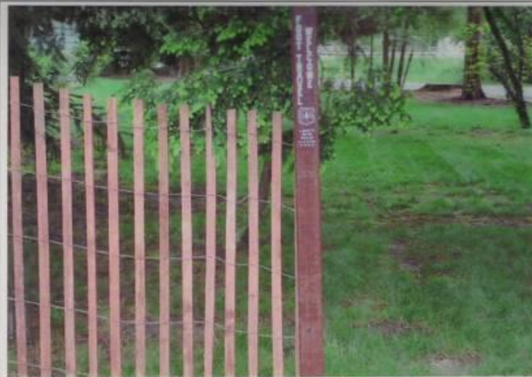
Option E: Lightweight wood fences and signs to prevent vehicle access to stream, walk-in camping allowed.
