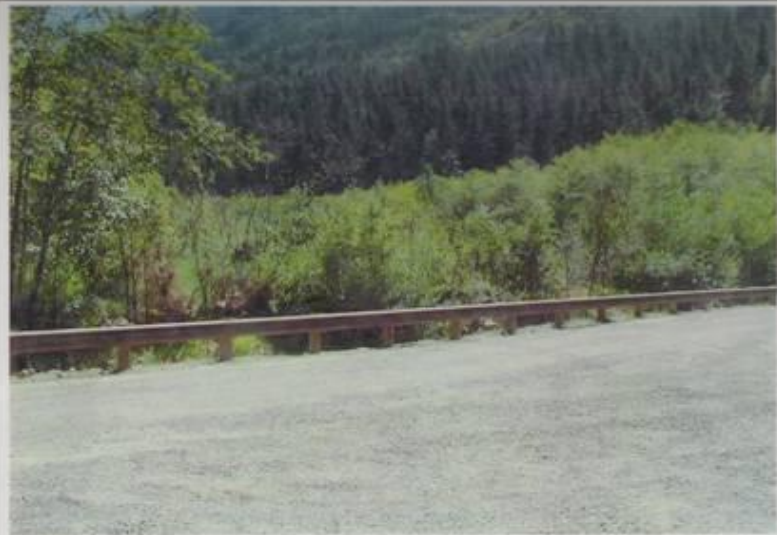
Option C: Guardrails to prevent vehicle access to stream, walk-in camping allowed.
