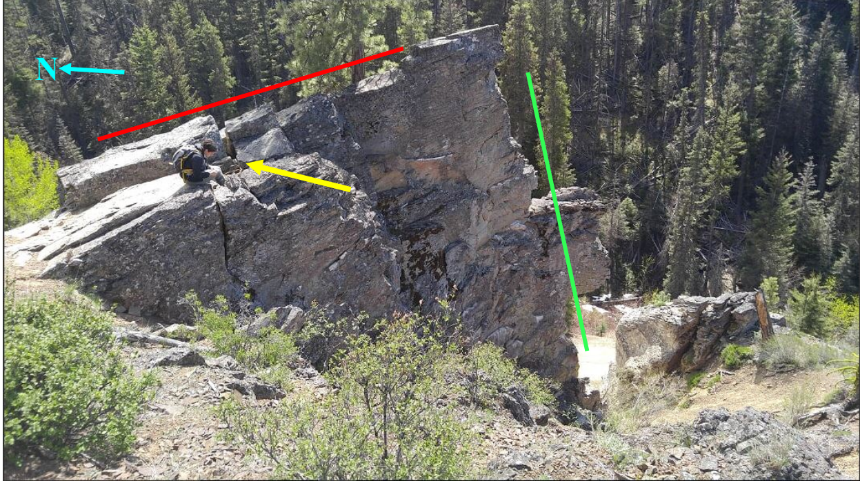
Figure 4. Anti-dip (Green) and dip slope (Red) of monolith at site HC1 (Fig. 10 shows location of this site). Myself taking trend and plunge measurements for scale (Yellow arrow). View SW. Daniel O'Dell photo.
