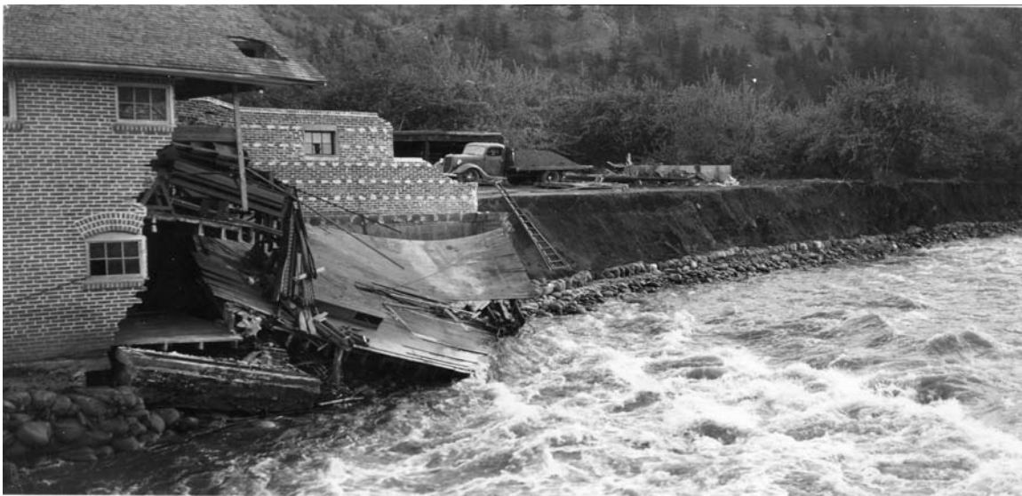
Figure 23. Pre-existing rock riprap bank protective structure located above river mile four during the 1948 flood (Photograph courtesy of the Wenatchee Valley Museum & Cultural Center, Gamble Collection, #83-28-10).
