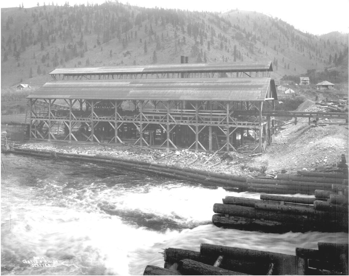
Figure 11. The Kellogg sawmill near Mills Canyon, 1914. Clearly, the Entiat River was heavily modified in this section. The millpond/reservoir behind the dam held vast quantities of timber and was hundreds of feet long (Photograph courtesy of the Washington State Historical Society, Asahel Curtis Collection, #30019).
