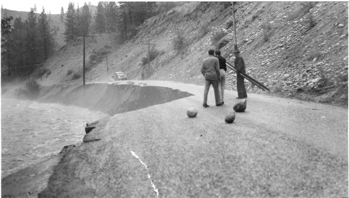
Figure 14. Flood damage to the Entiat River Road near the Stanley Grade, 1948. (Photograph courtesy of the Wenatchee Valley Museum and Cultural Center, Gamble Collection, #83-28-7).
