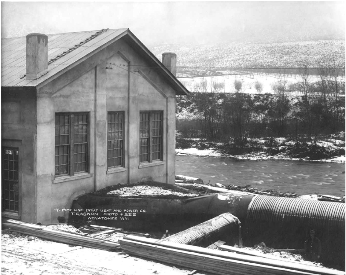
Figure 10. Power plant built by the Entiat Light and Power Company near river mile one, ca. 1910. The large pipe in the photograph funneled water impounded by a three-foot high dam located more than a mile upstream (Photograph courtesy of the Wenatchee Valley Museum and Cultural Center, Chamber Collection, #86-24-90).
