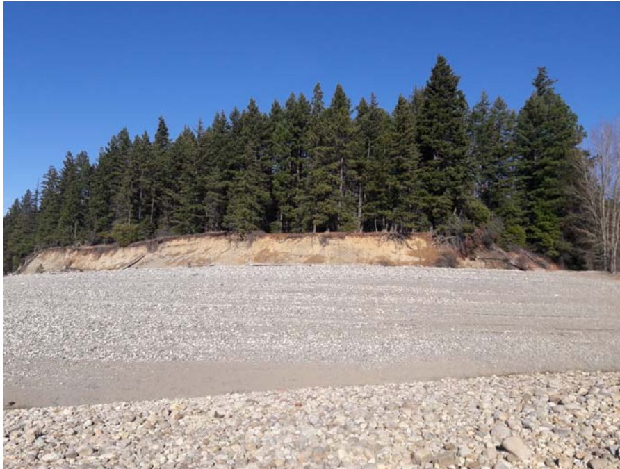
Figure 22: Bluff erosion near Sandelin Lane, Cle Elum Lake. Bluff eroded in Quaternary Evans Creek alpine glacial drift. Varial zone in the foreground. View towards the east. Photograph by Michael Horner, June 2019.
