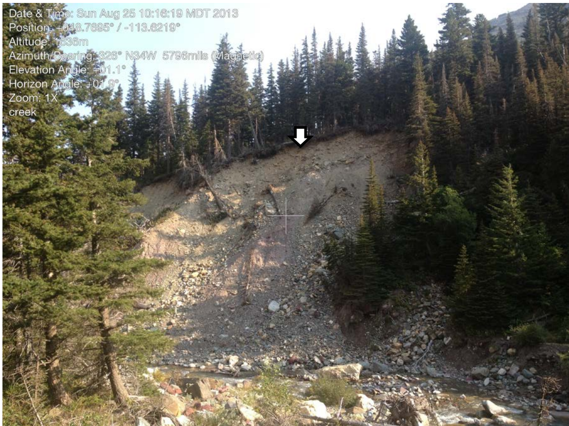
Figure 20. Linear scarps indicating a translational slide along Canyon Creek on the Cracker Lake Trail. Photo by author.
