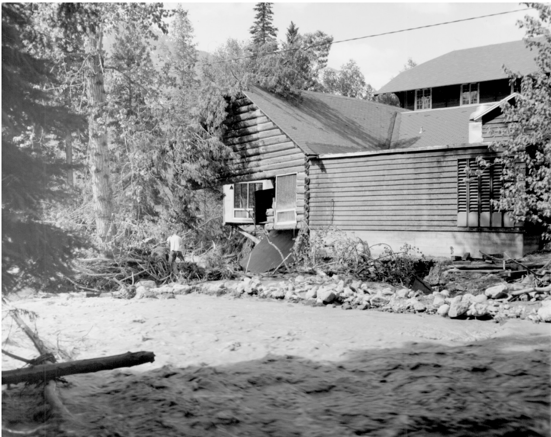
Figure 5. Snyder Creek following flood stage near Lake McDonald Lodge in Glacier National Park, spring 1964. Note damage to the dining room from flooding. National Park Service archives, June 9, 1964, John J. Palmer photographer.
