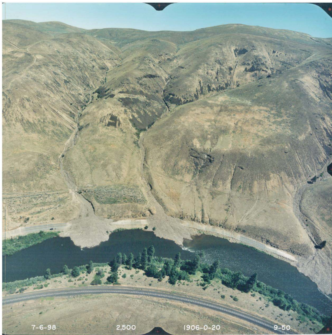
Figure 1. Debris flows covering State Route 821 from the 1998 thunderstorm event. Photo from Washington State Department of Transportation, South Central Office.
