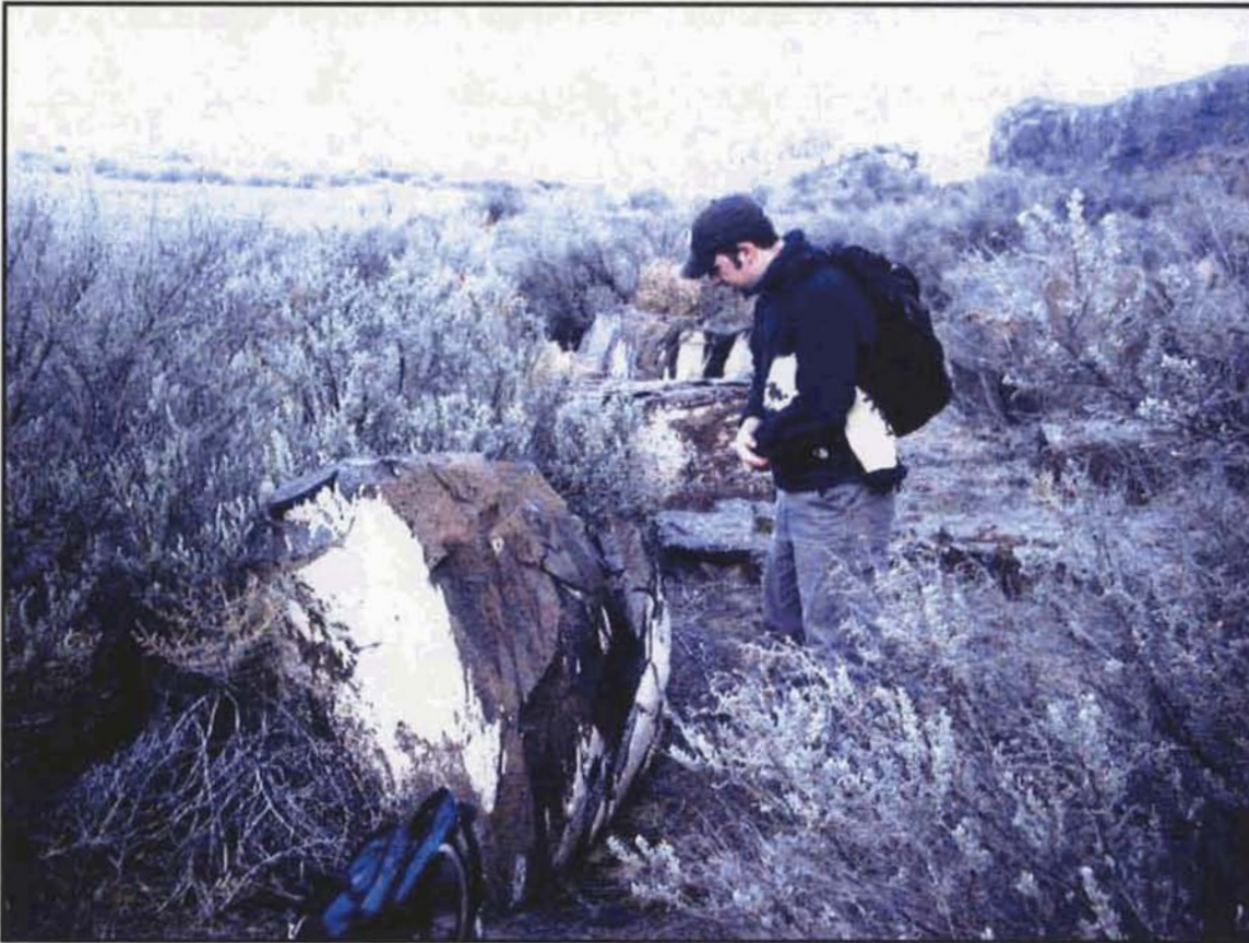
Figure 20. Oblique ground view of spalling, basalt corestone resting in fosse of pendant bar located on the south side of the Ancient lake cataract. Note the jointing parallel to the surface on the rock creating a round corestone. Also note the red-brown weathering rind and white evaporite coating. (Seth Mattos for scale)
