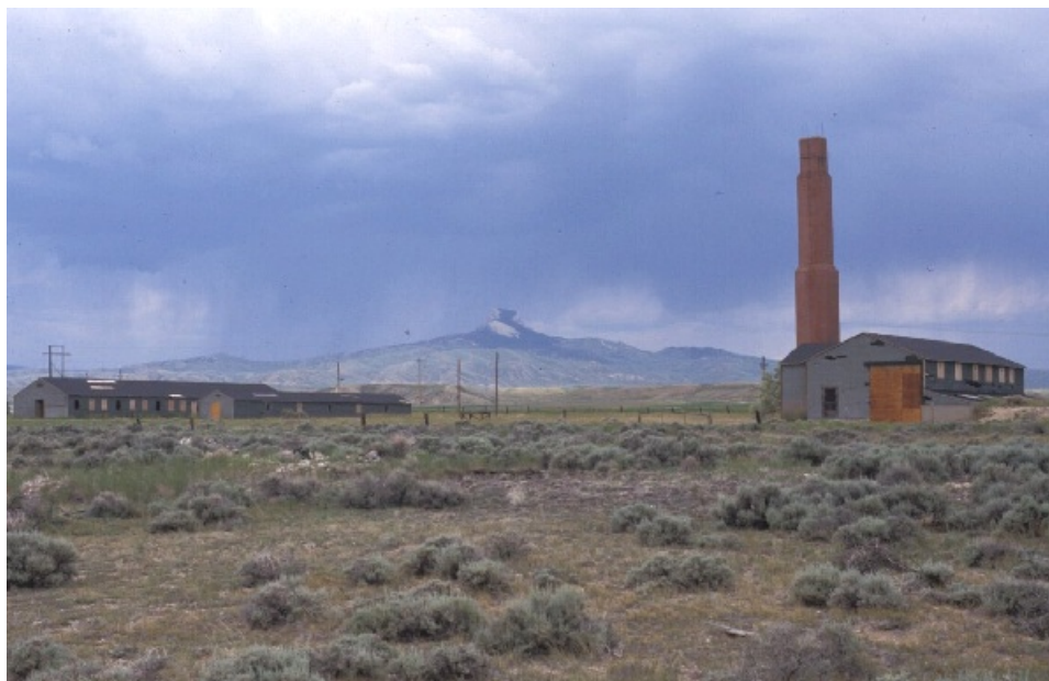
Figure 4.28. Former hospital heating plant, Heart Mountain Relocation Center. Author photograph, June 2003.
