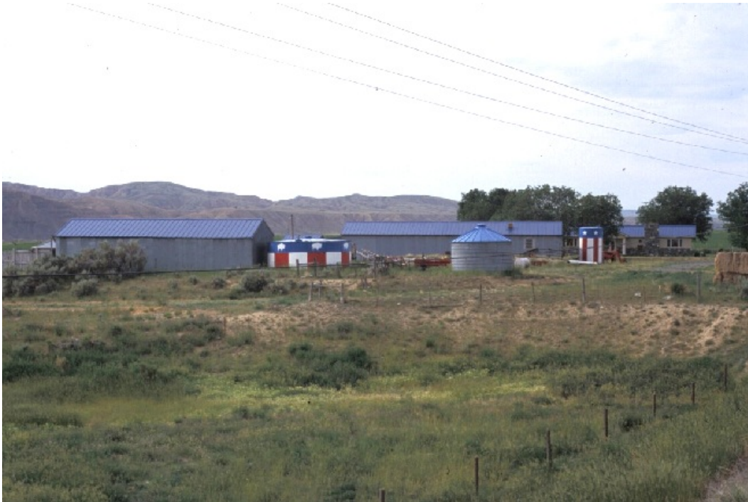
Figure 4.26. Remains of barracks on farm near former Heart Mountain Relocation Center. Author photograph, June 2003.
