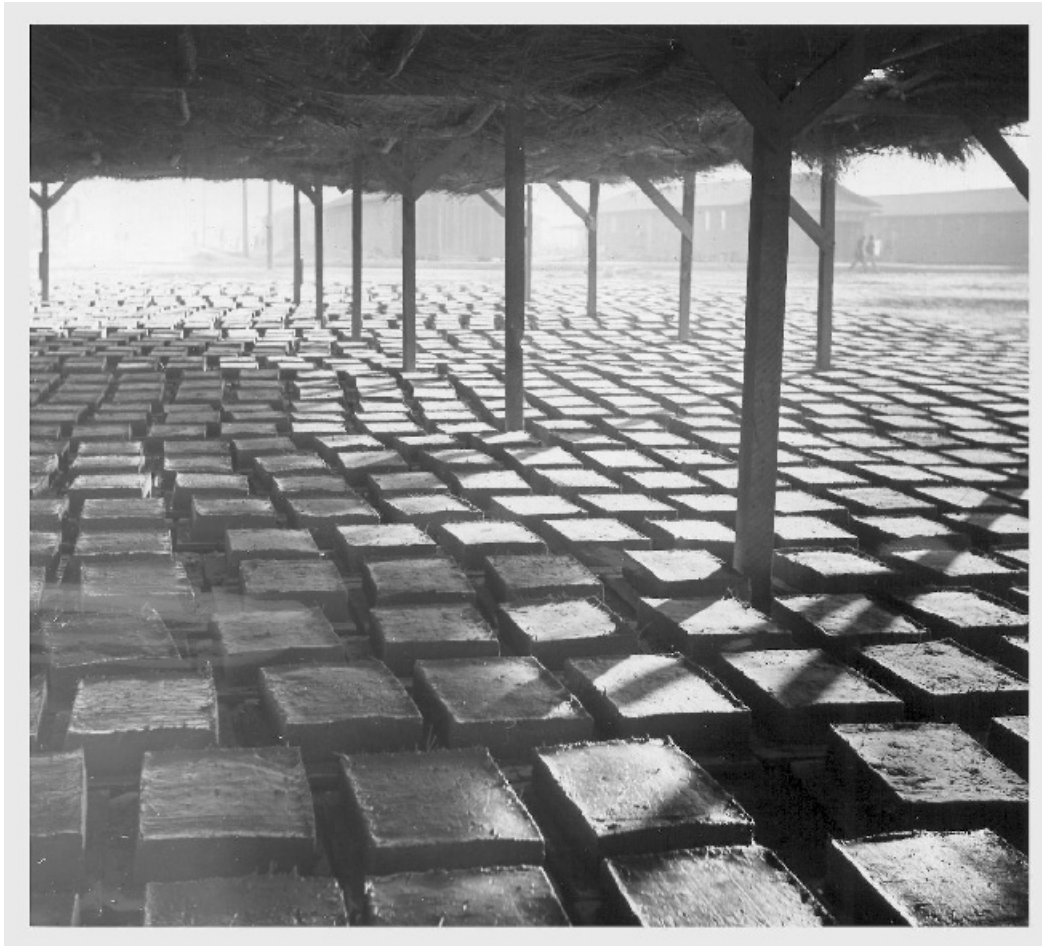
Figure 9.21. Adobe bricks drying at Poston Relocation Center. Francis Stewart photograph, December 1943. Courtesy of the Bancroft Library, University of California, Berkeley. Volume 2, Section A, WRA # A-821, War Relocation Authority Photographs of Japanese-American Evacuation and Resettlement, Series 1: Colorado River Relocation Center, Poston, Arizona.
