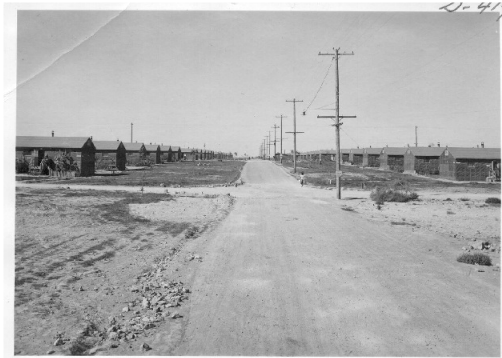
Figure 5.14. View down a Minidoka street. Note the grass planted between the road and the barracks, and the barracks garden on the left. Unknown photographer, August 1943. Courtesy of the Bancroft Library, University of California, Berkeley. Volume 25, Section C, WRA # G-414, War Relocation Authority Photographs of Japanese-American Evacuation and Resettlement, Series 9: Minidoka Relocation Center, Hunt, Idaho.
