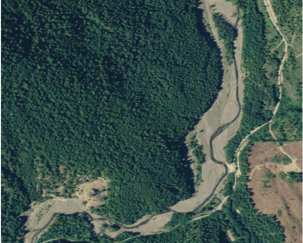
Figure 29. Aerial photograph of Cabin Creek near the mouth of Cole Creek showing the near-stream disturbance zone ranging from 200-500 ft (60-150m) in width.
