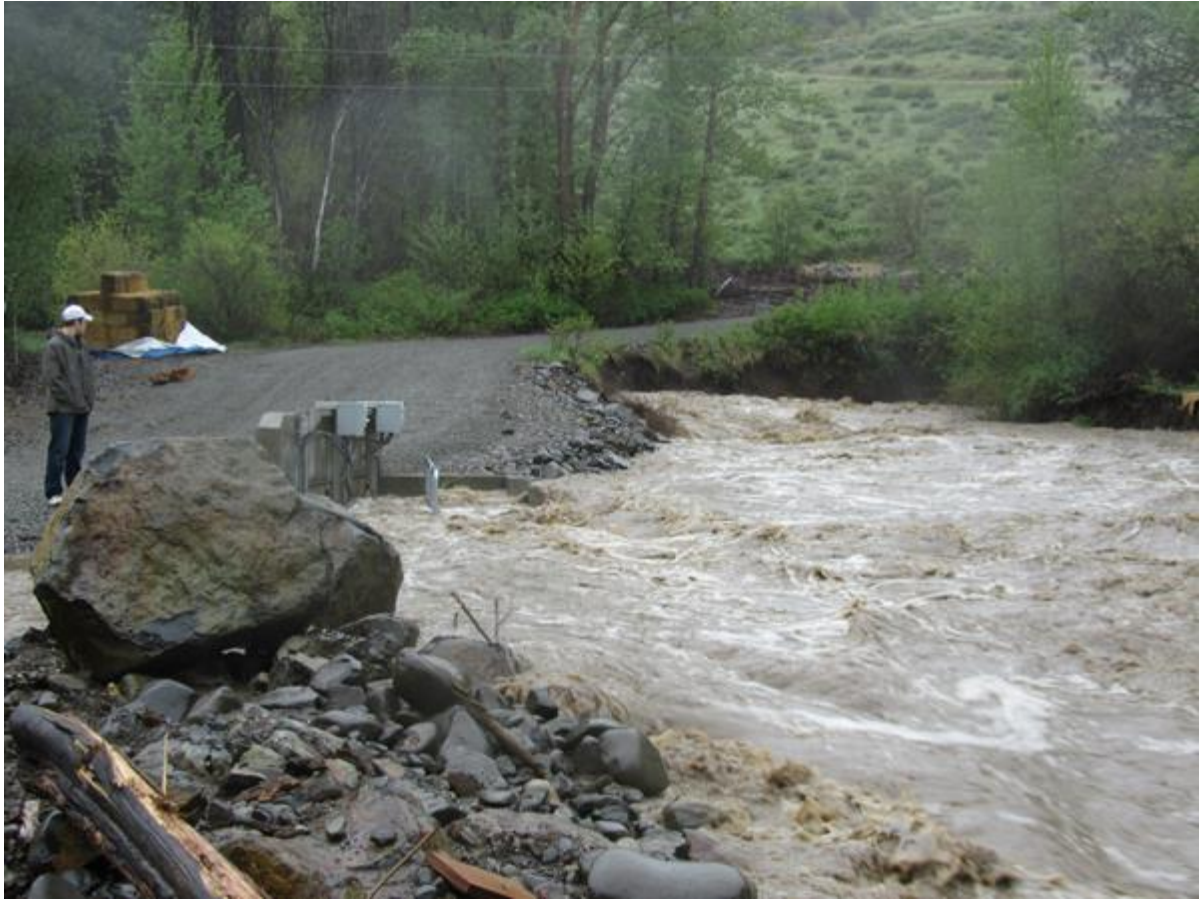
Figure 6: The large flood of May 15, 2011, near the intake to the Taneum irrigation canal. Photo taken by Paul Tappel, 2011.
