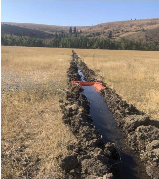
Figure 2. Spreading ditch enhancement
