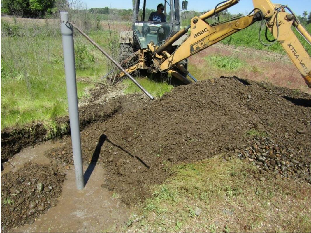
Figure 10. Initial installation of monitoring wells. A larger pipe was used to protect the well and filter fabric wrapped around it during installation. Note the high water table that did not allow digging below a meter in gravel areas.
