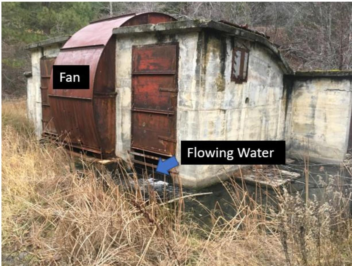
Figure 38. A picture of the fanhouse. The fanhouse is a groundwater overflow point for the Roslyn Mines located on the Suncadia property directly east of the Cle Elum River.
